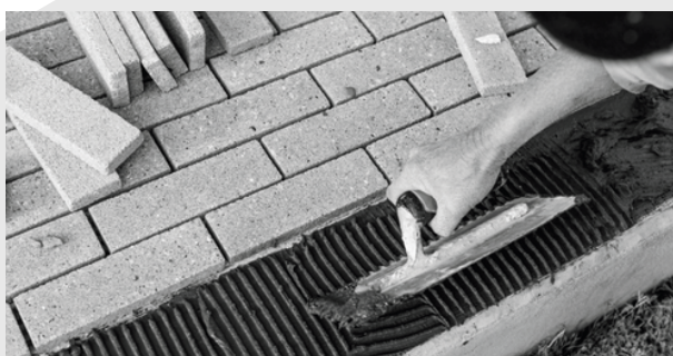
Apply mortar to substrate, screed with the notched trowel.
